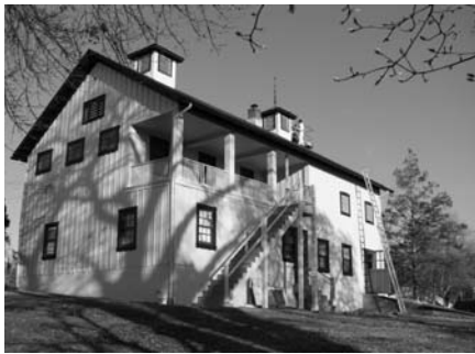
The Carriage House on the Manor grounds
