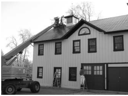
Special equipment was brought in for painting.
