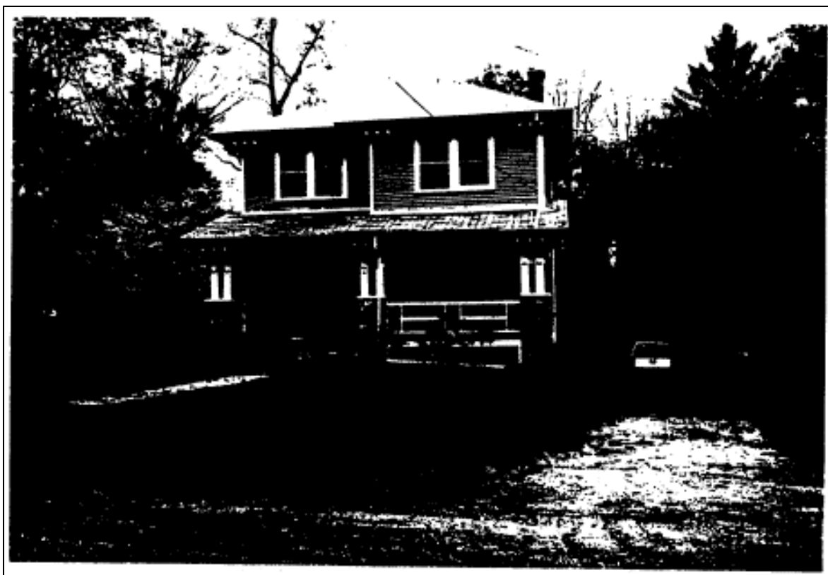
Figure 26: Photograph of 3922 Washington Street.
