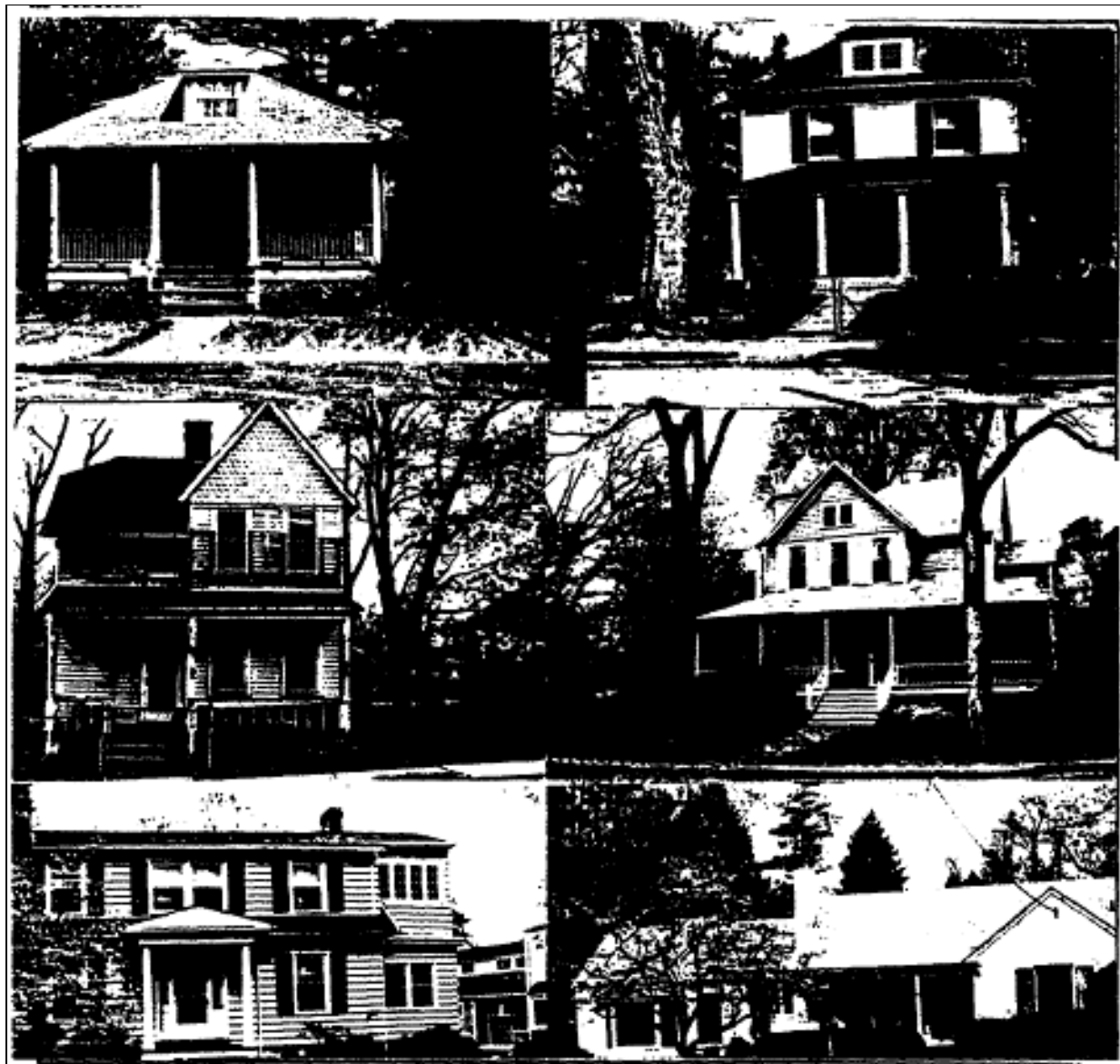
Figure 10: Scale and Building Height in Kensington structures in the district are 2 stories in height and 45% are two-and-one-half stories.
